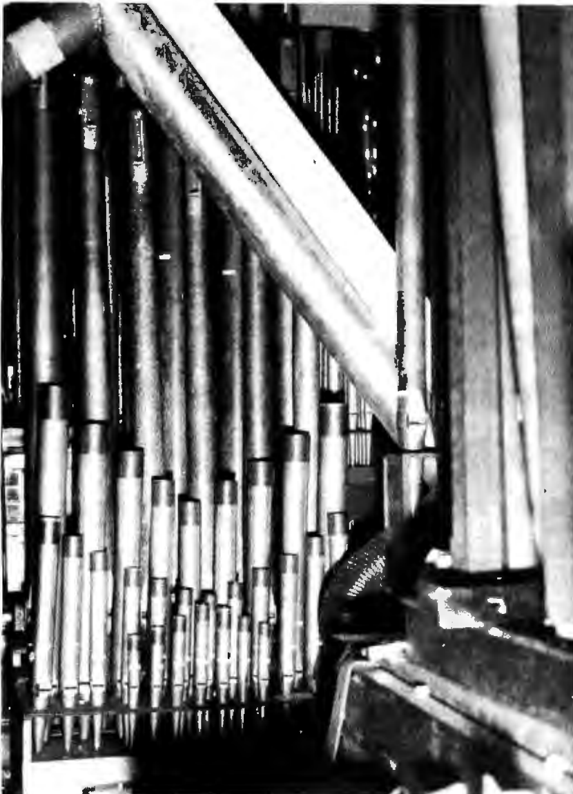
Photo 3: Another view of the organ showing the swell chest and echo chest.
